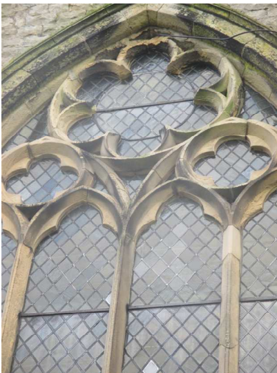
North window masonry
