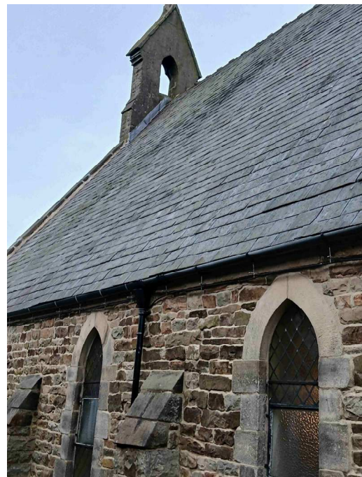
The repaired roof
